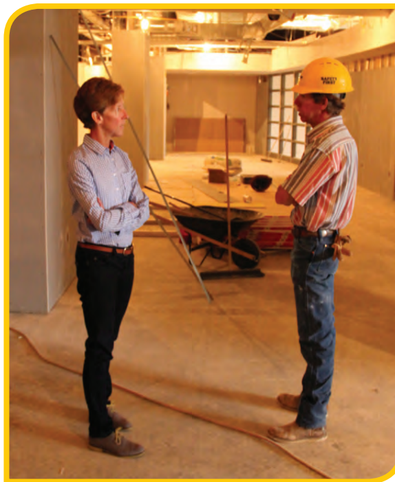
CCC President Dr. Becky Rowley discusses the Phase VI project with Brian Bunce of Stoven Construction.
